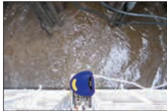
EchoSonic II level transmitter shown in lift station application.
